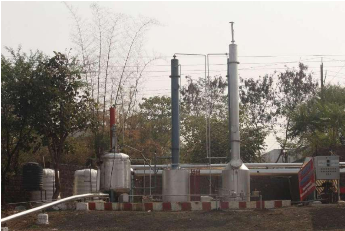
Figure 1: CCS Plant at RKDF University
